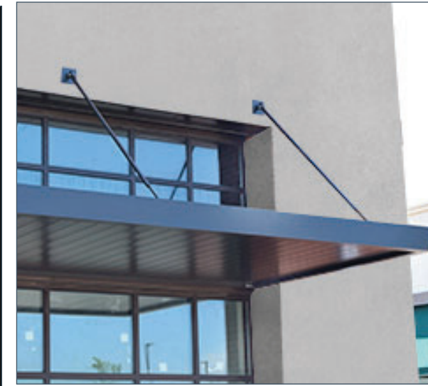
7 METAL CANOPY Manufacturer: General Contractor Finish: Painted Steel Tube Color: DE 6385 Black Bean By: Dunn Edwards
