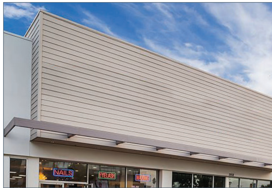
2 HARDIE BOARD SIDING Manufacturer: Hardie Board Model: Artisan Siding, V-Groove Siding ( Primed for Paint ) Color: DE 6376 Looking Glass, Dunn Edwards
