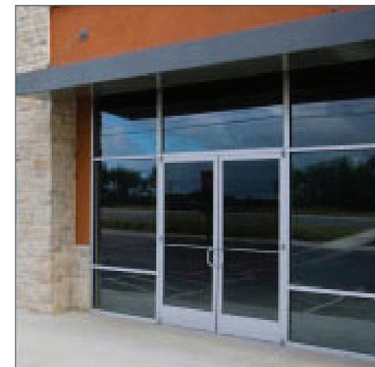
4 STOREFRONT Manufacturer: Arcadia Finish: #11 / Clear AC-2 STOREFRONT GLASS Manufacturer: PPG Color: 1" Clear Float Glass
