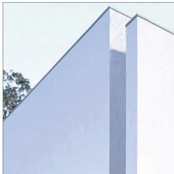
1 STUCCO Manufacturer: Highland Stucco Smooth Steel Trowel Paint Color By Dunn Edwards A, B & C
