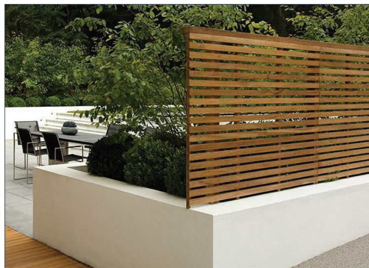
5 WOOD SLATS (PATIO AREA) Manufacture: By General Contractor Finish: Natural Wood - Architectural Grade Color: Cedar Naturaltone ST-533 - BEHR Premium Semi Trans. Waterproofing Stain/Sealer
